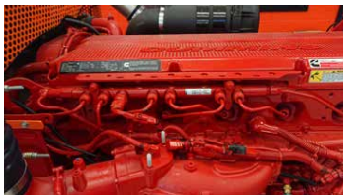
Cummins CRD rail
